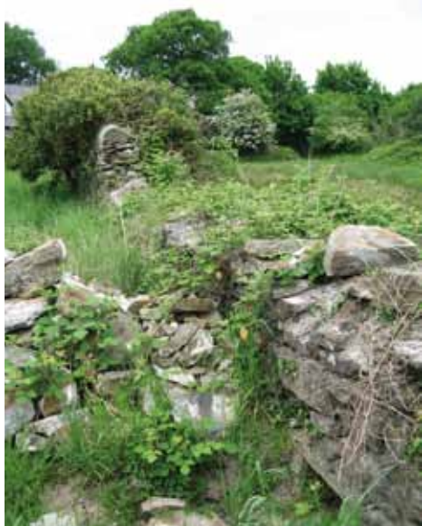
Groeswen Chapel wall transformed from this...
